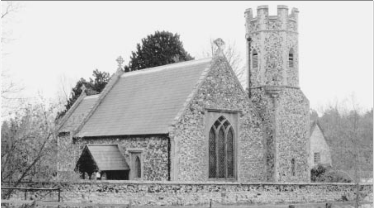
West Tofts church from the west
